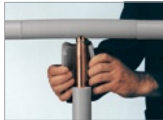
2. Attach the preformed part
