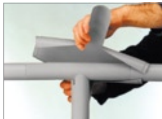
4. Attach the outer shell of the preformed part
