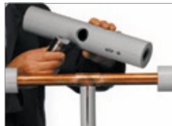
4. Cutting a hole with the punch
