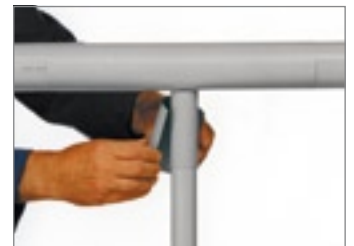
6. Sealing the joints
