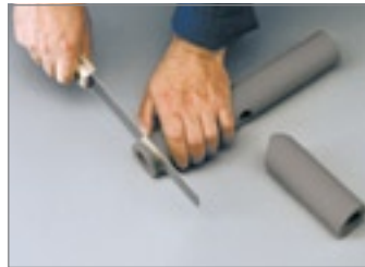
1. WICU® preformed parts are used for the subsequent insulation of T-pieces up to 28 mm
