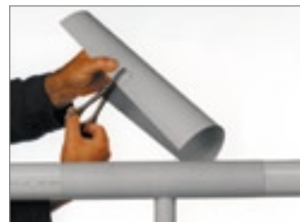
5. Cutting the outer shell to size
