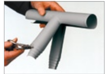
3. Cut the outer shell of the preformed part
