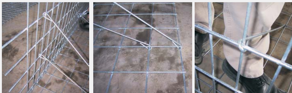
Fixing of the restraining hooks
