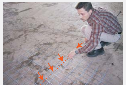
Inserting the plug-in lock
