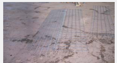
Preparation of front and bottom grid
