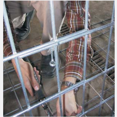
Overlapping and fixing of adjoining elements
