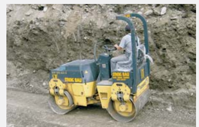
Compaction of the subgrade
