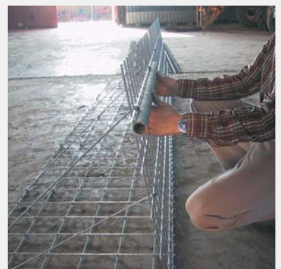
Temporary stiffening (e.g. steel pipe)
