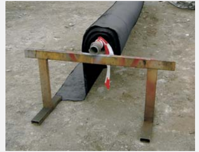
Cutting off the geosynthetic
