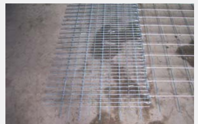
Installation of inner grid (if necessary)
